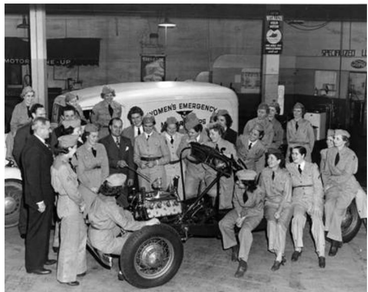
Red Cross Motor Corps Women receive training from Ford on the fine points of the Flathead V-8 engine.
